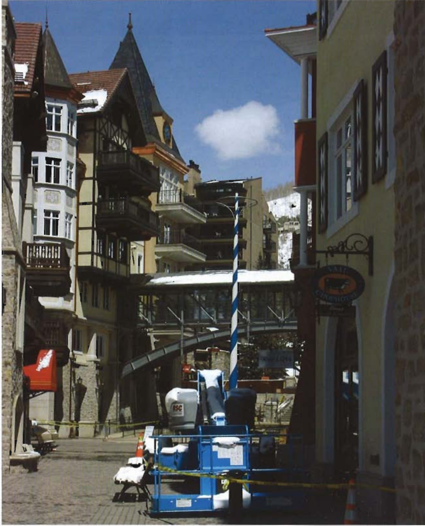
MOST OF THE PROJECTS ARE SCHEDULED TO BE COMPLETE IN 2010.
